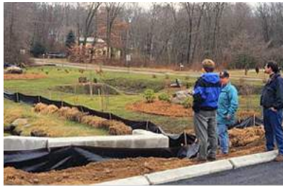
Construction reviewers periodically inspect construction sites to ensure that contractors have installed and maintained their erosion and sediment controls properly (Source: University of Connecticut Cooperative Extension System, 2000)
