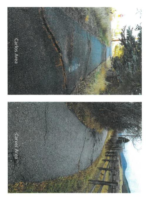
Tree roots undermining the trail – - Require complete removal of pavement (both), - Removal of roots (Carver) or
