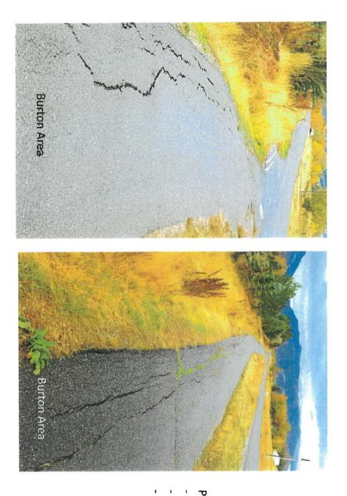
Pathway slumps (Burton Area) -- Require pavement removal - Additional fill and compaction
