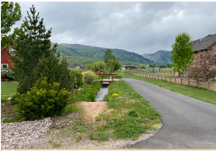
Looking towards location of new diversion structure
